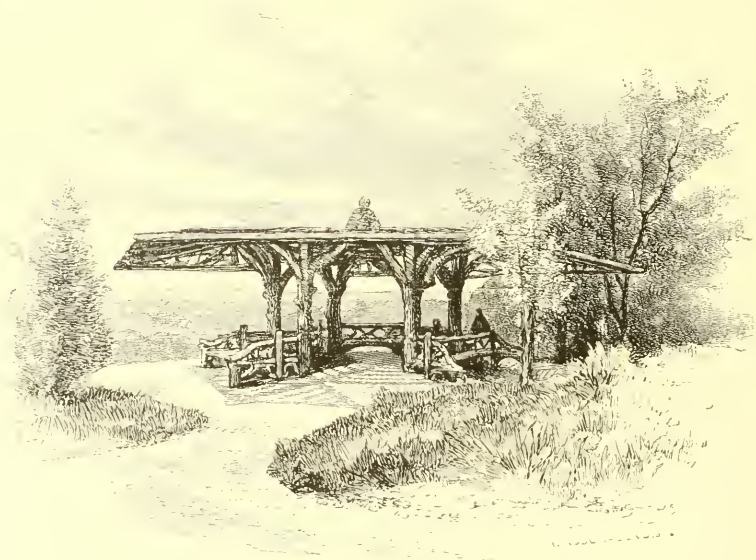
SUMMER-HOUSE IN RAMBLE NEAR THE BELVEDERE.
